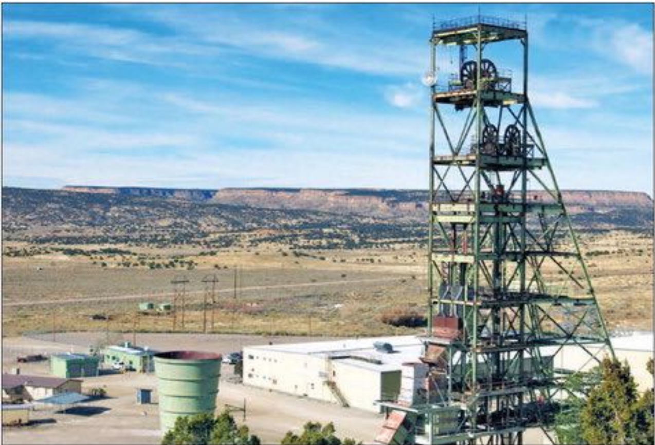
An overview of the Mount Taylor Mine surface facilities and 24-foot headframe above the mine shaft are visible in this 2015 photo.
